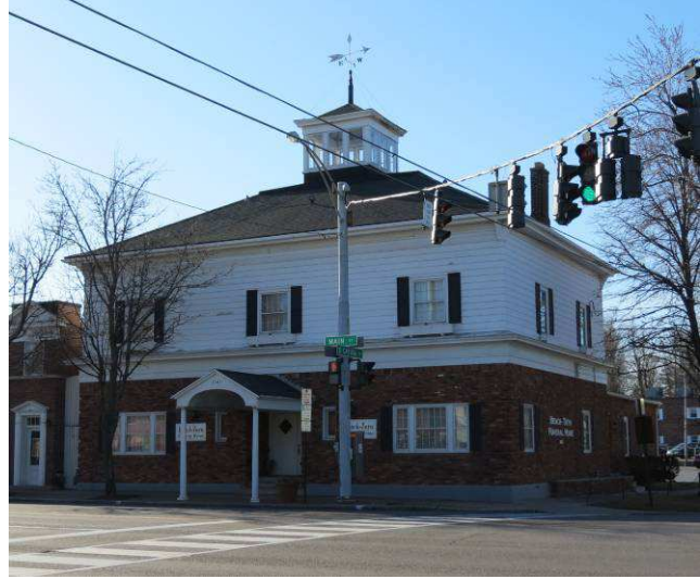
Photo 4.9 5541 Main Street Built in 1888 and significantly altered, this building is a large scale example of an Italianate commercial building, retaining its large rectangular massing, hipped roof and cupola.
