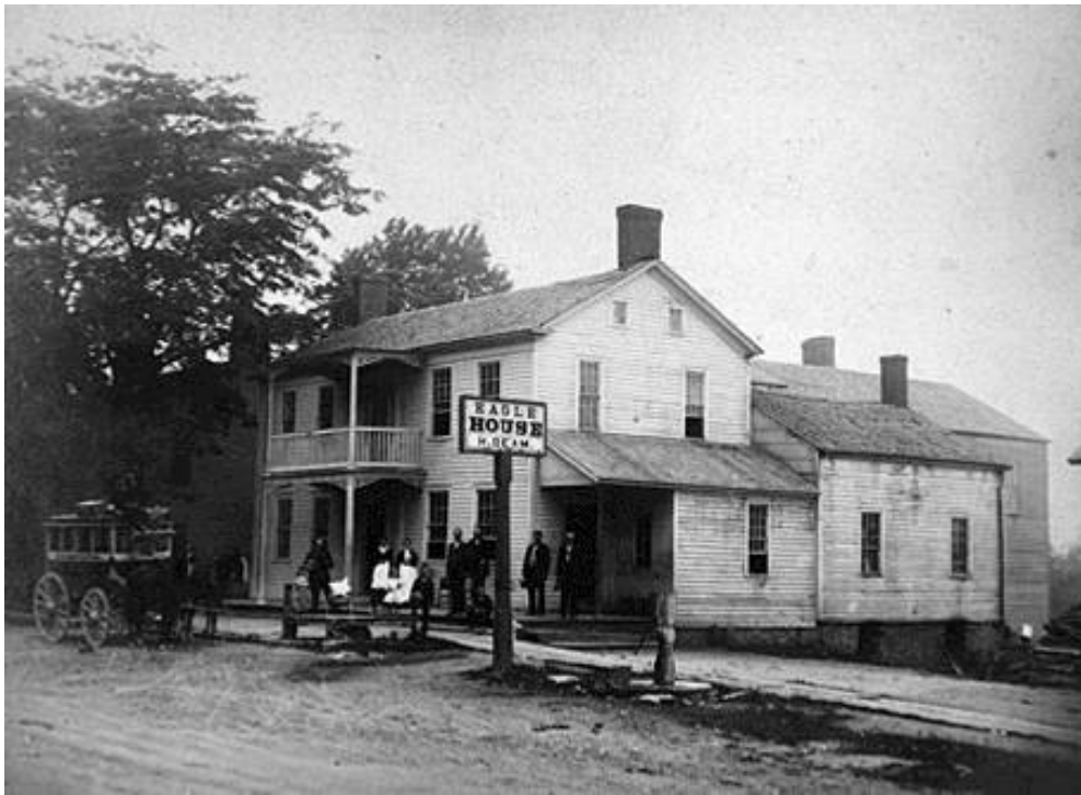
Fig 3.2 The Eagle House at 5578 Main St (ca. 1900s view)
