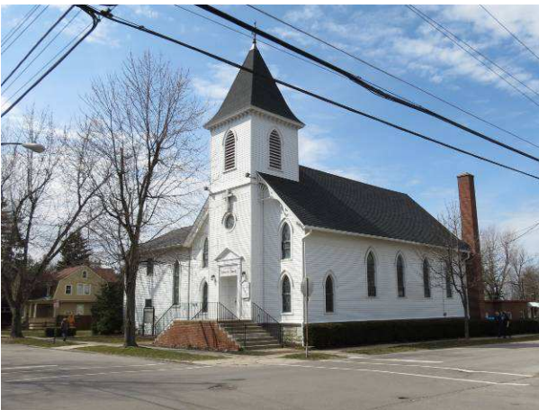
Photo 4.18 68 Eagle Street St. Paul's Evangelical Lutheran Church, built in 1900, is a good example of a vernacular Gothic Revival wood-frame church building.
