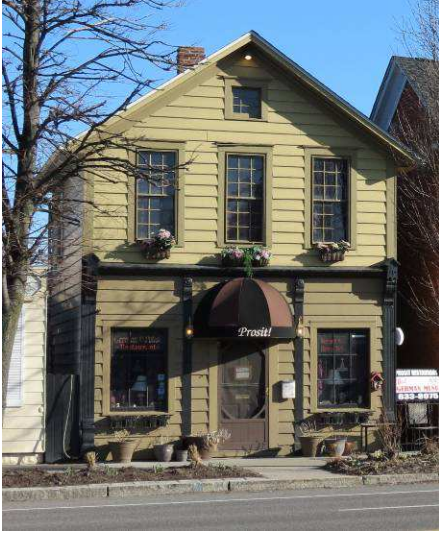
Photo 4.8 5428 Main Street Reflecting the influence of the front-gabled Greek Revival design, this building retains an excellent cast iron Italianate-style storefront.
