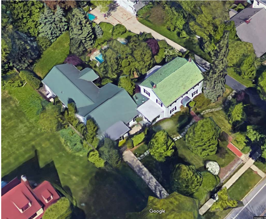
Image #1: Aerial view from Google Maps. Lighter green roof is the original house and darker green roof is a large addition constructed in 2004.
