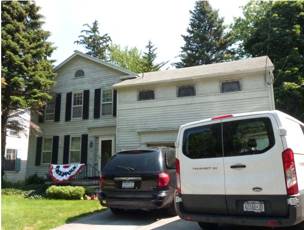
Photo #1: Looking northeast
