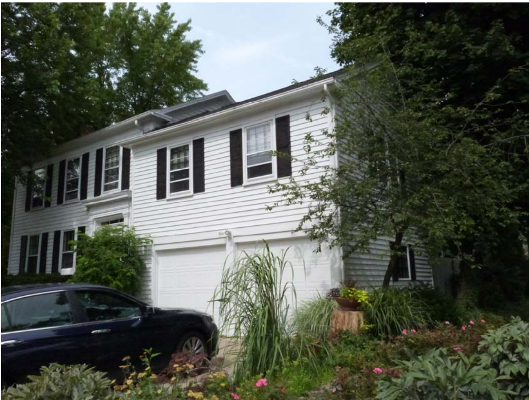
Photo #2: Looking northeast
