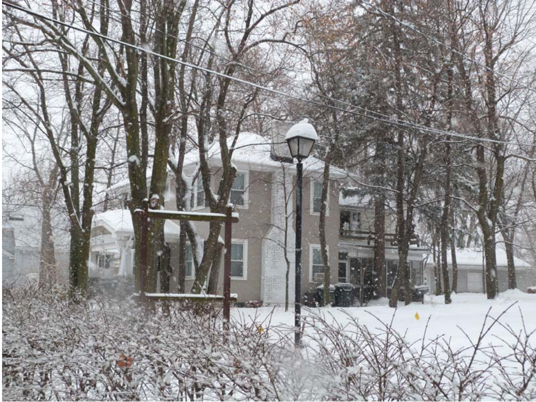
Photo #3: Looking northeast from adjacent property. Note porch and older portion of house, as well as older barn/carriage house, at rear.
