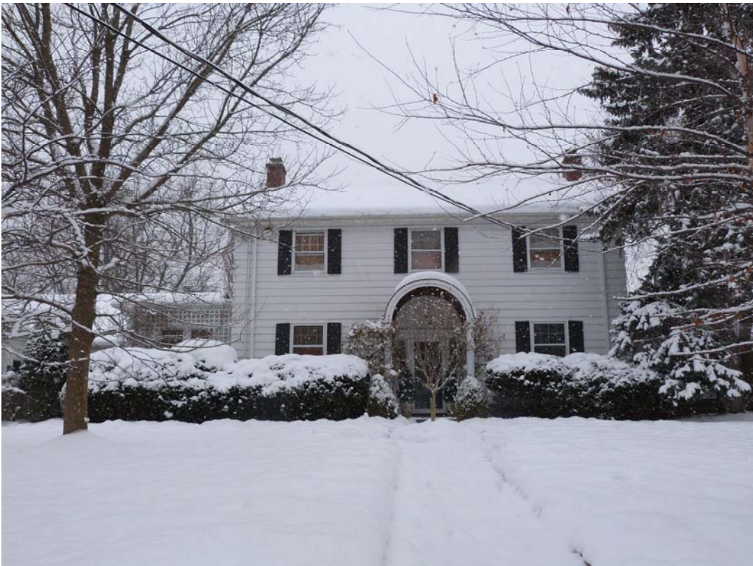
Photo #2: Looking west, clearer view without vegetation
