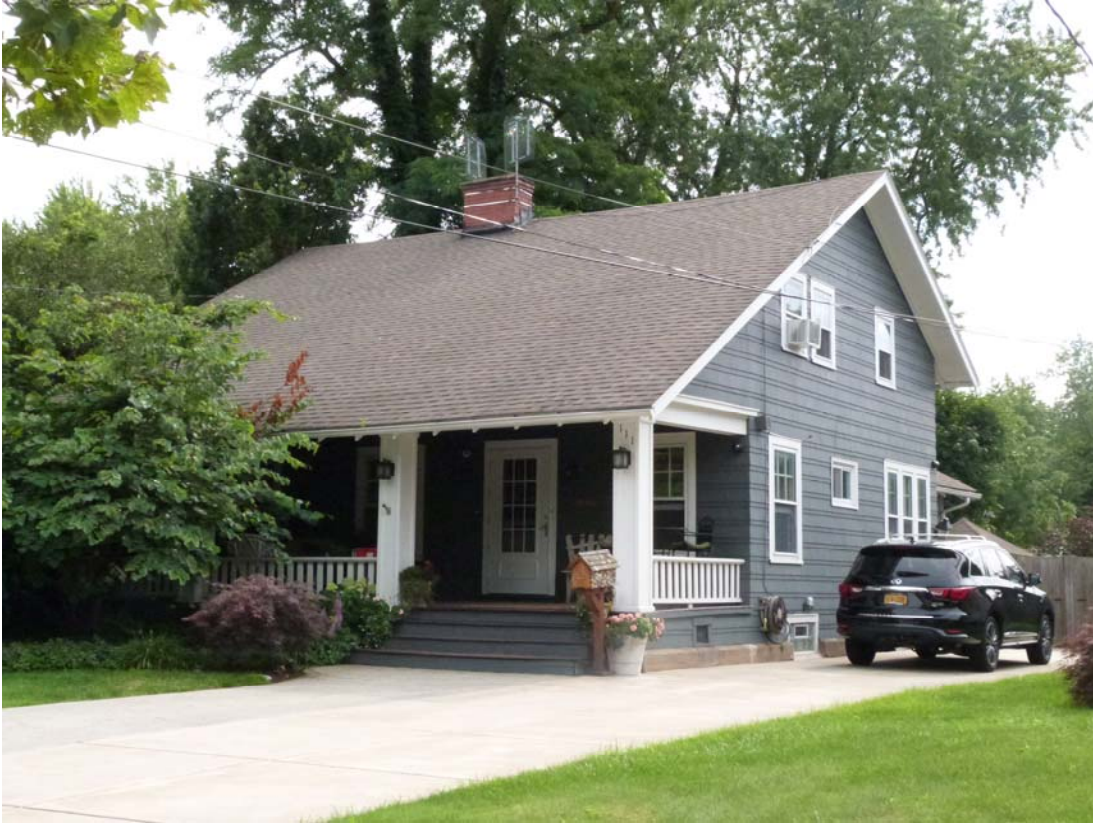
Photo #1: Overview looking southwest
