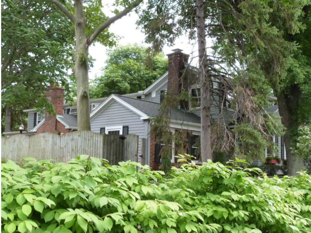
Photo #3: Overview looking southeast
