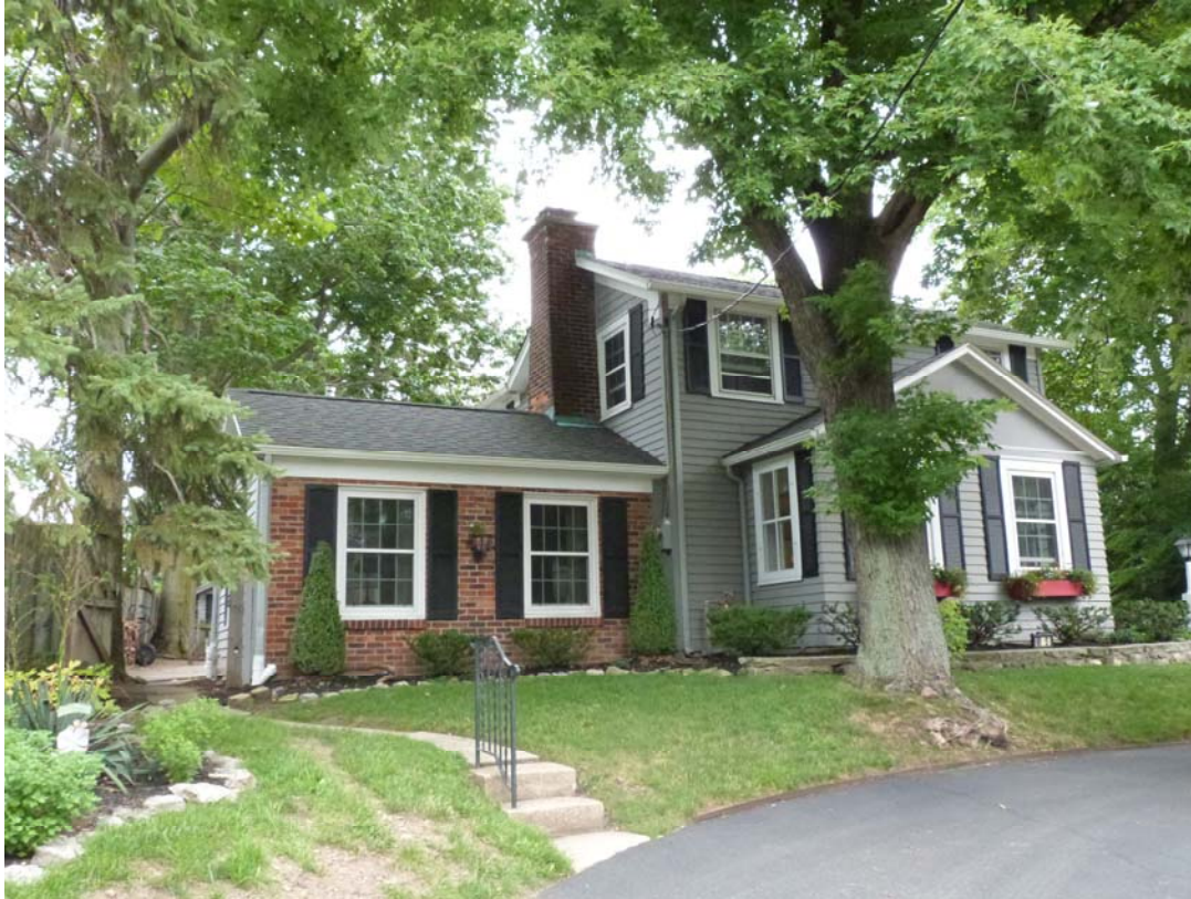
Photo #1: Looking southeast
