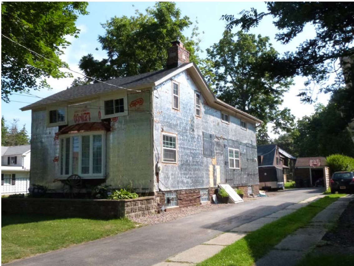
Photo #4: Looking northeast during exterior alterations, taken early August 2017
