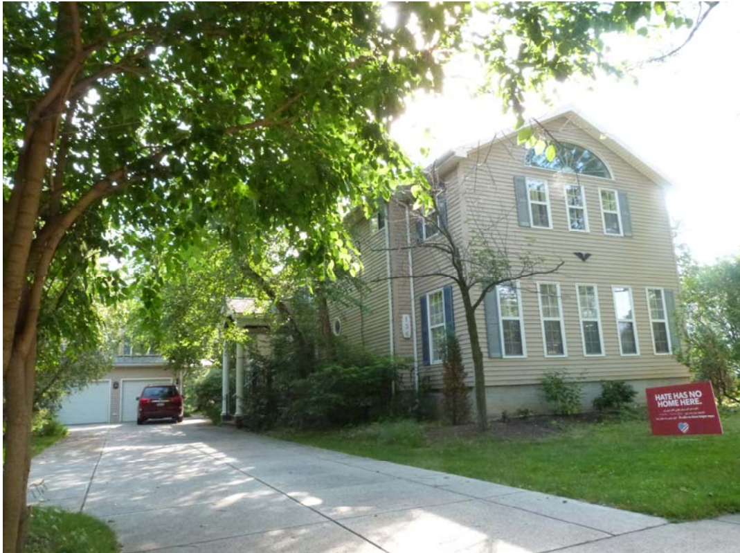
Photo #1: Overview looking southeast
