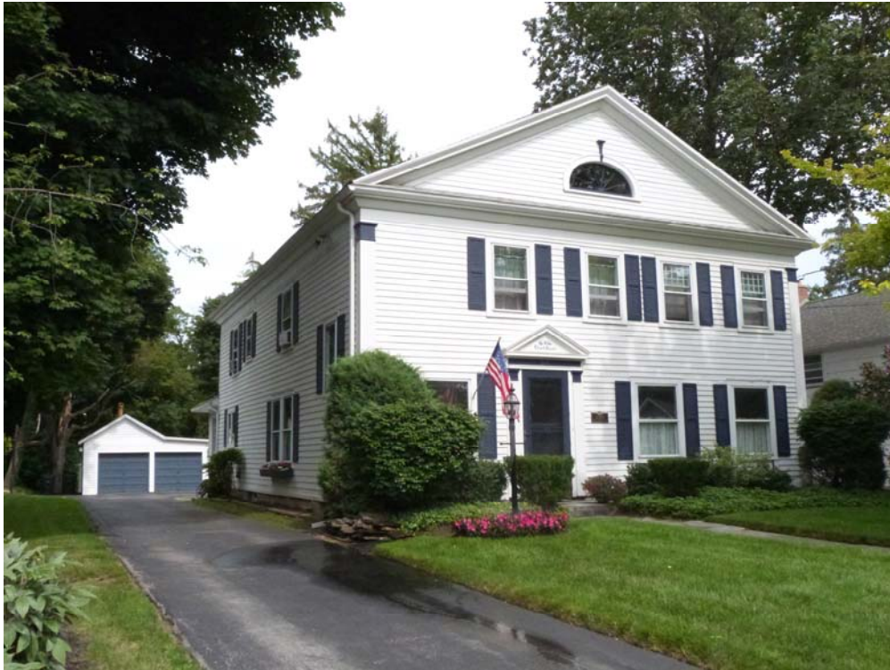
Photo #3: Looking southeast
