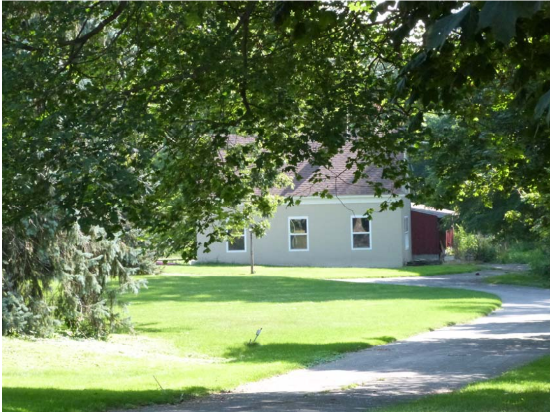
Photo #2: Looking west from S. Cayuga Rd. toward barn on property, which was historically associated with adjacent house at 204 S. Cayuga Rd.
