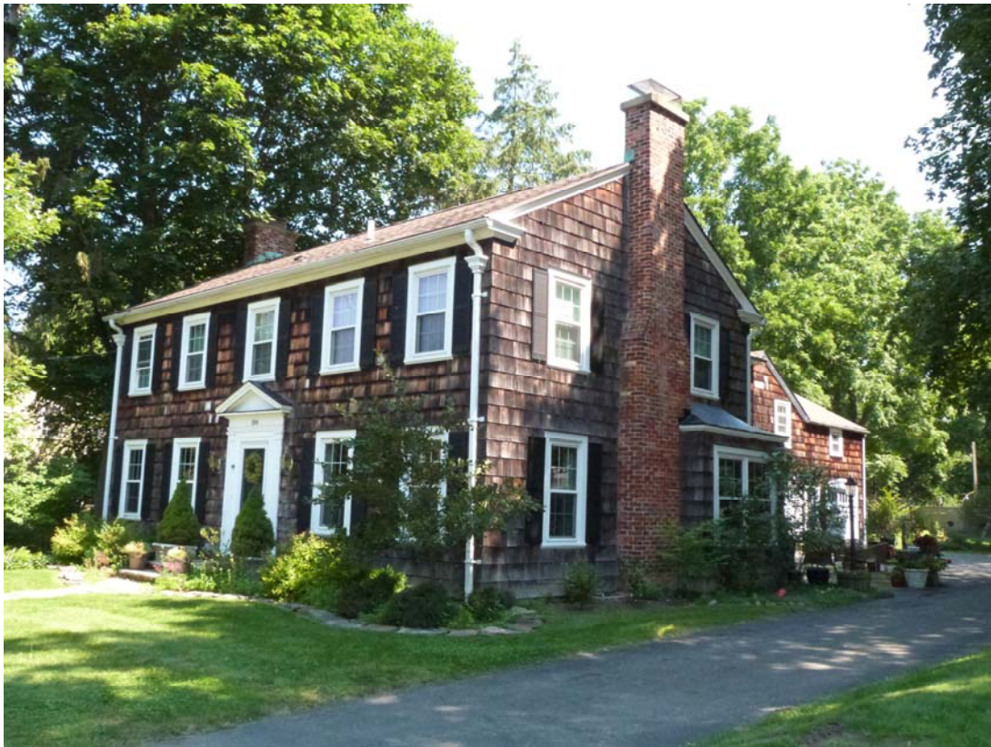
Photo #2: Looking northeast
