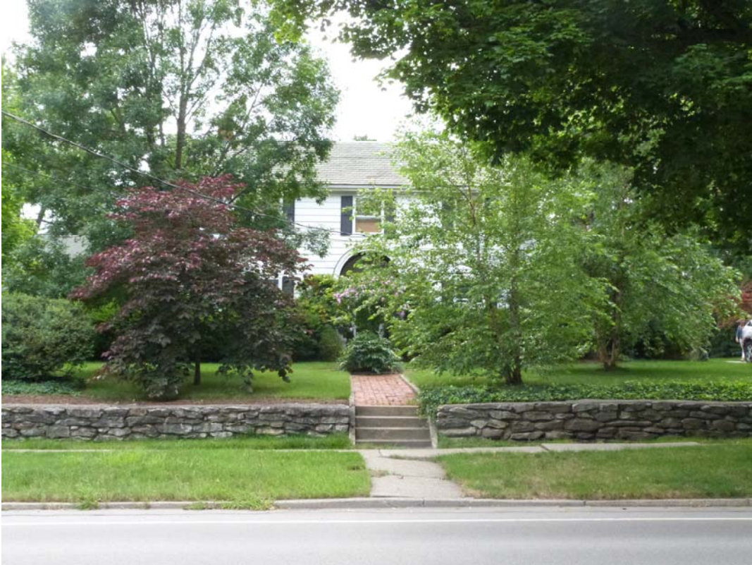
Photo #1: Overview looking west
