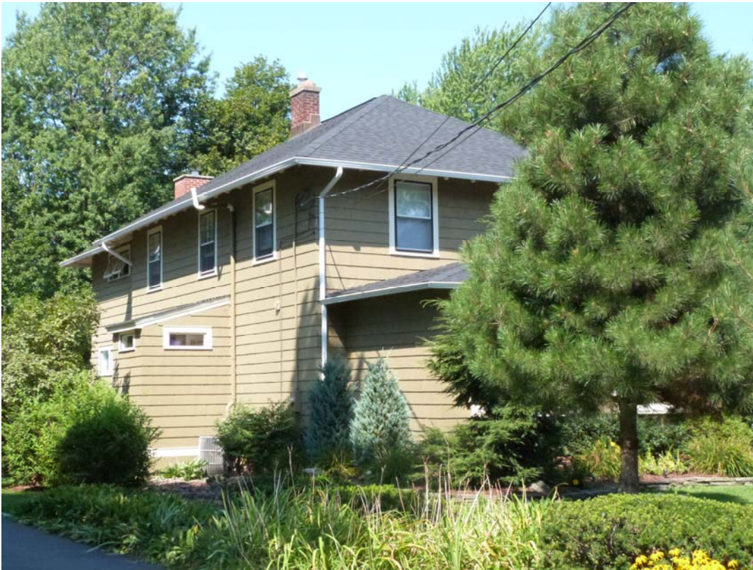
Photo #2: Looking northwest
