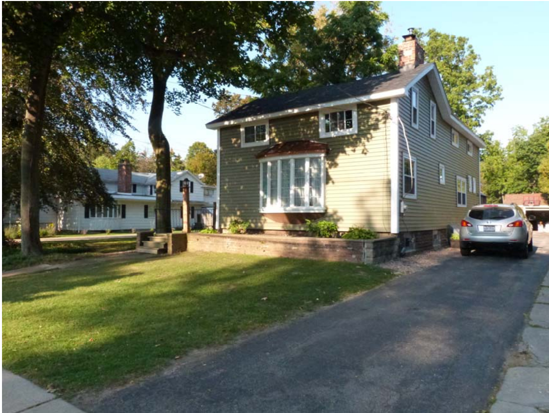
Photo #1: Overview looking northeast, mid-September 2017
