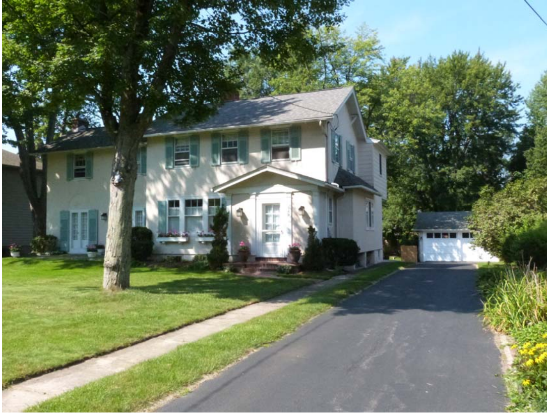
Photo #1: Overview looking southwest
