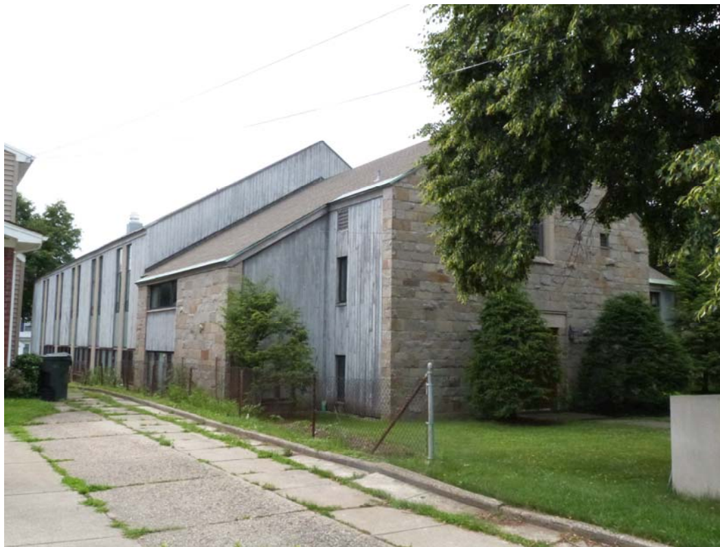
Photo #4: Looking northwest toward rear (south) side of Education Building
