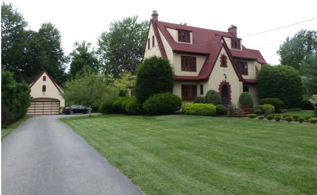
Photo #1: Overview looking northwest
