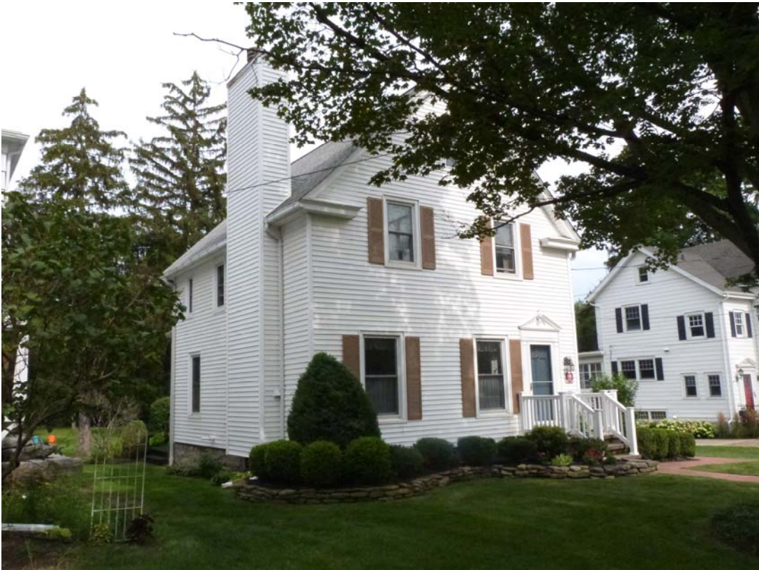
Photo #2: Looking southeast
