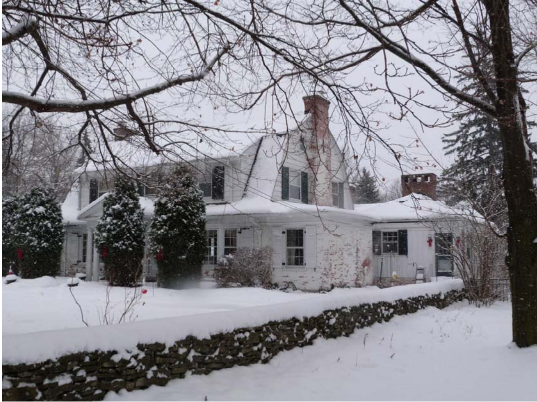
Photo #3: Looking southwest from S. Cayuga Rd.
