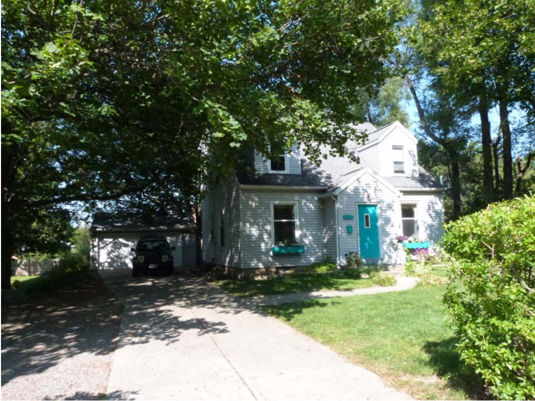
Photo #1: Overview looking west
