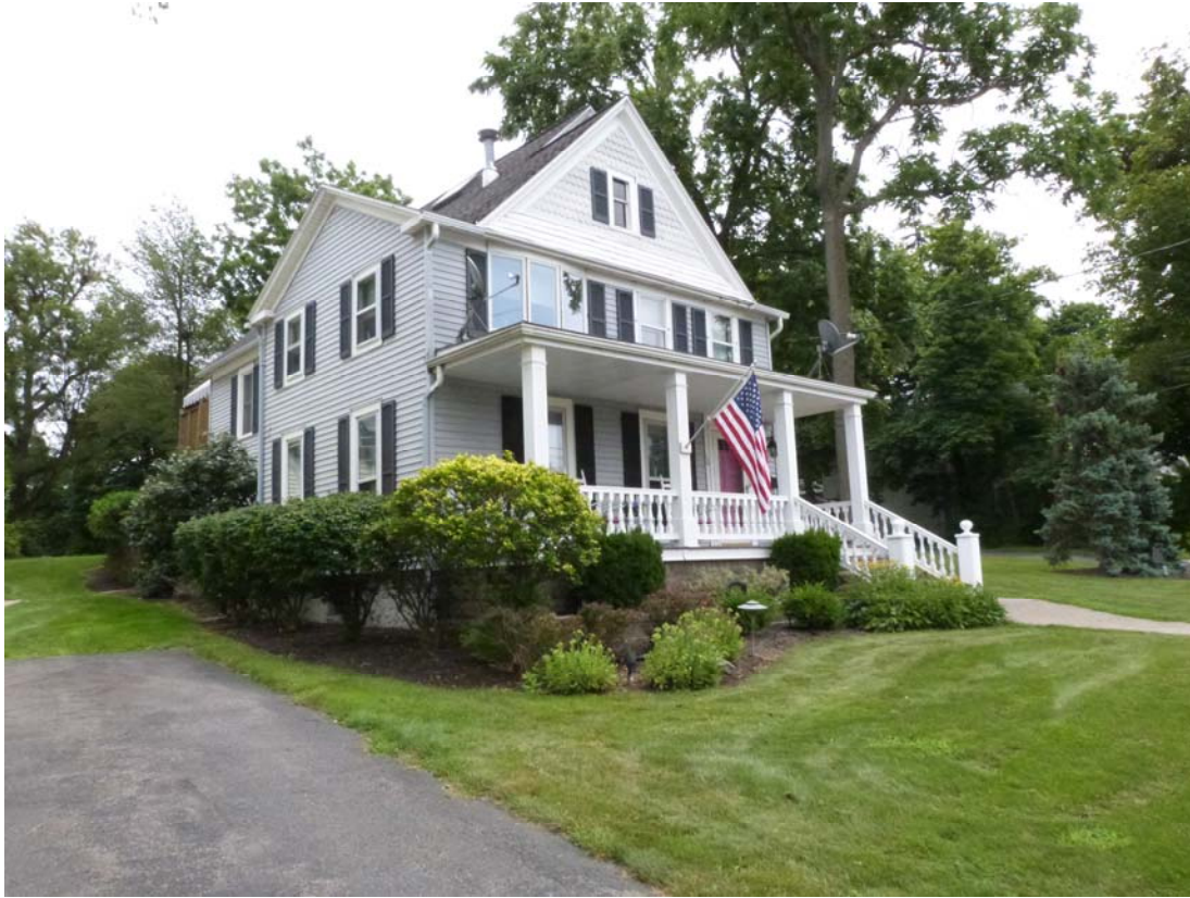
Photo #1: Looking southeast
