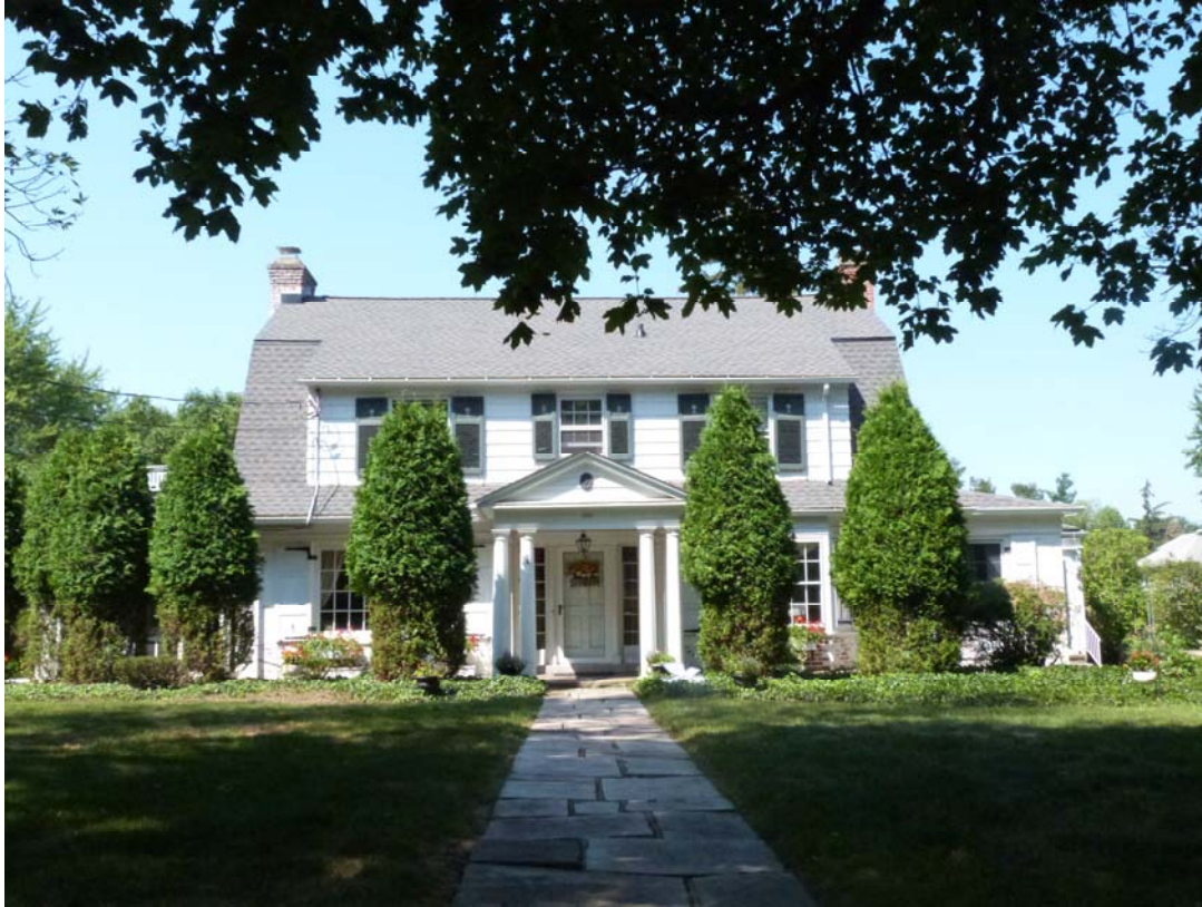
Photo #1: Looking west from S. Cayuga Rd.
