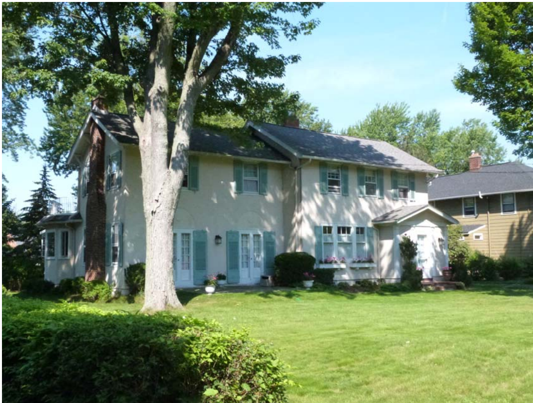
Photo #2: Looking northwest
