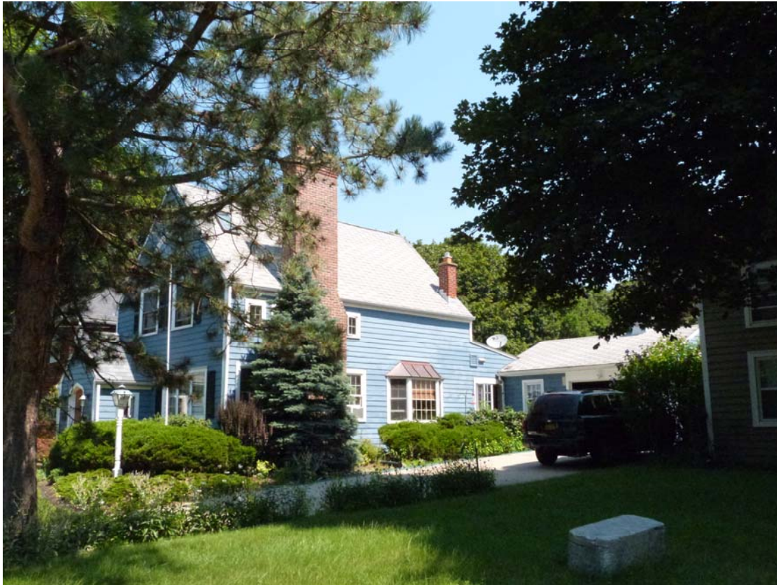
Photo #3: Looking northeast from adjacent property
