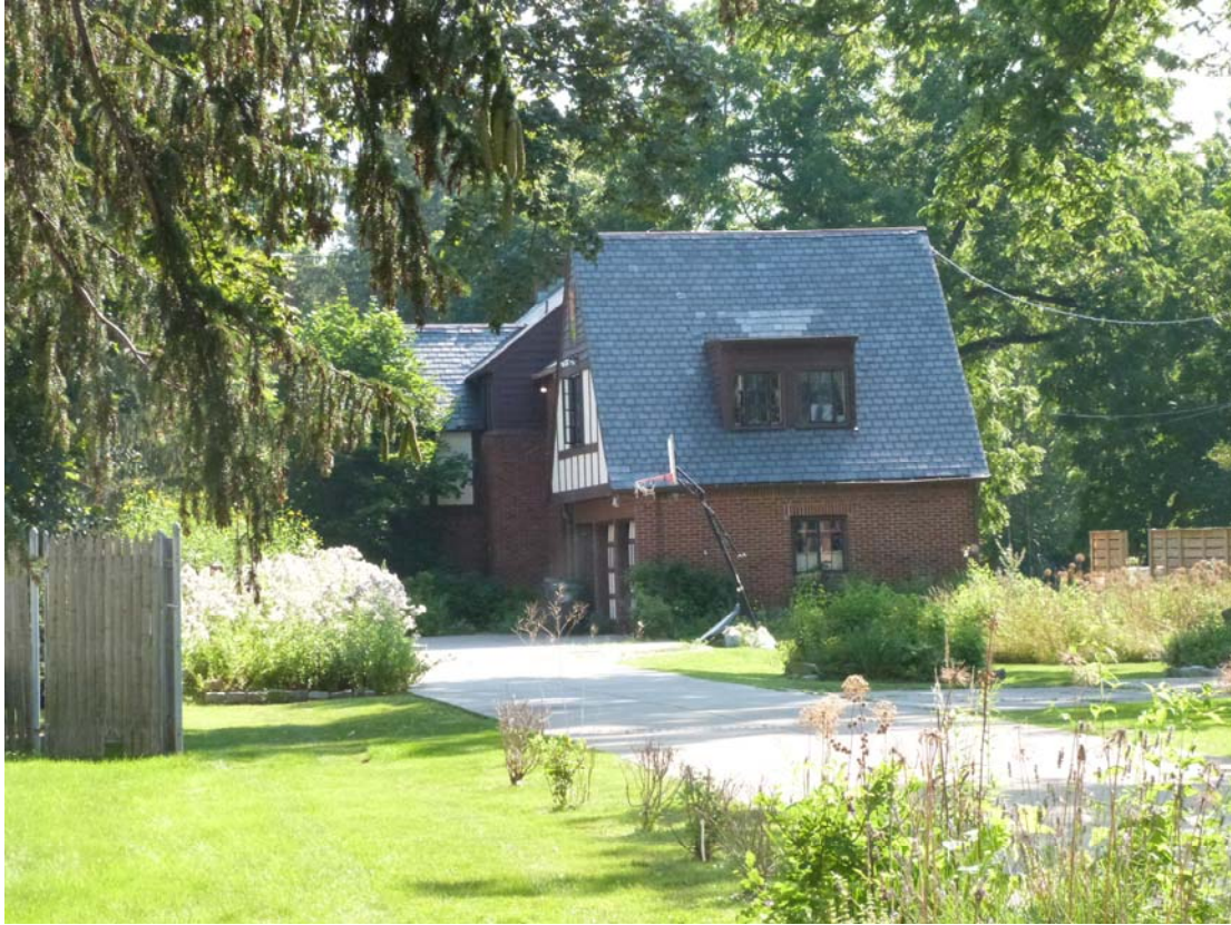
Photo #1: Looking southeast
