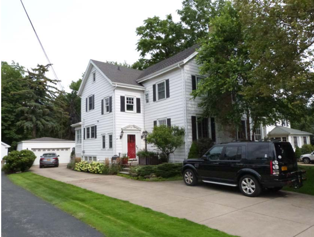
Photo #1: Overview looking southeast
