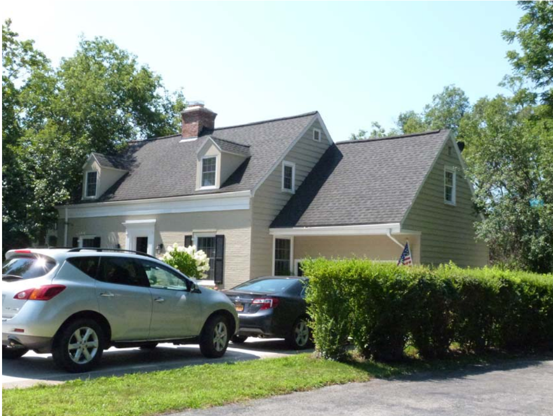
Photo #2: Looking southwest
