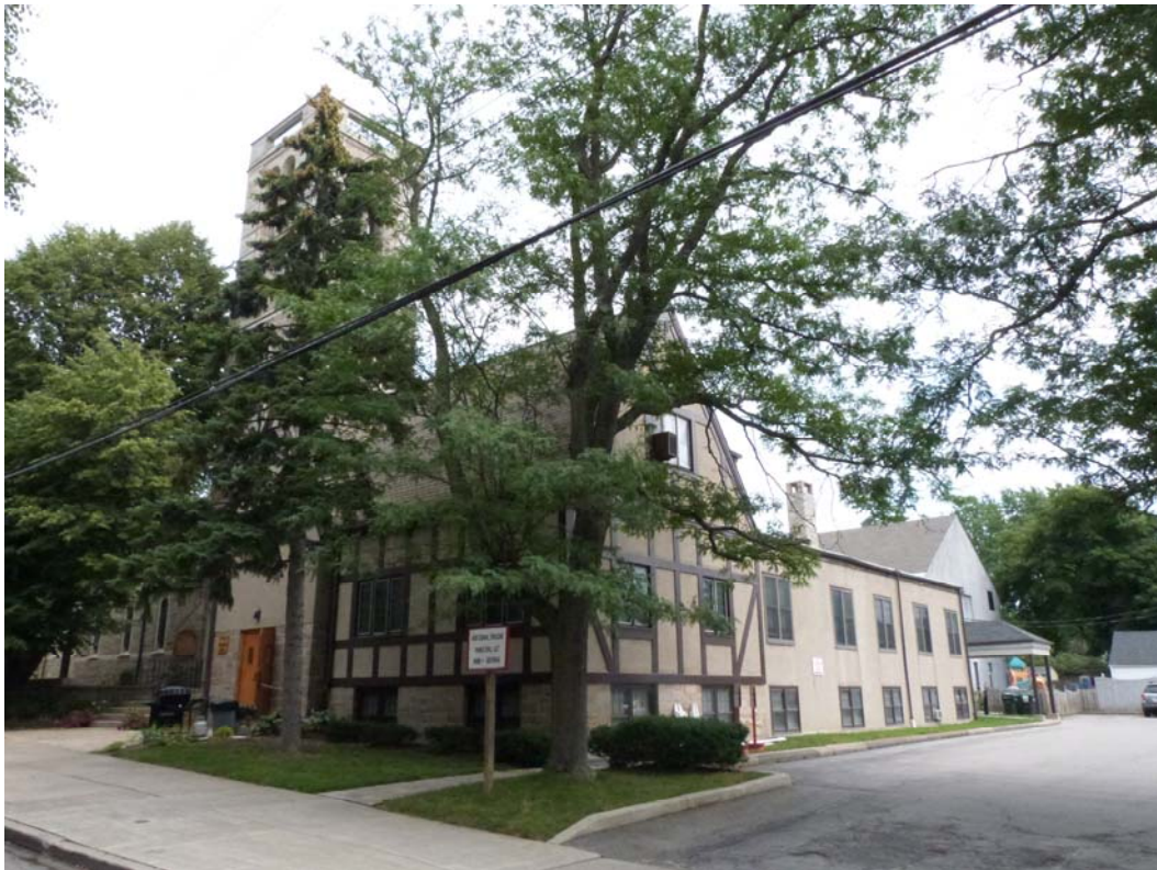
Photo #2: Looking southeast toward rear of church and parking lot accessed from Milton St.
