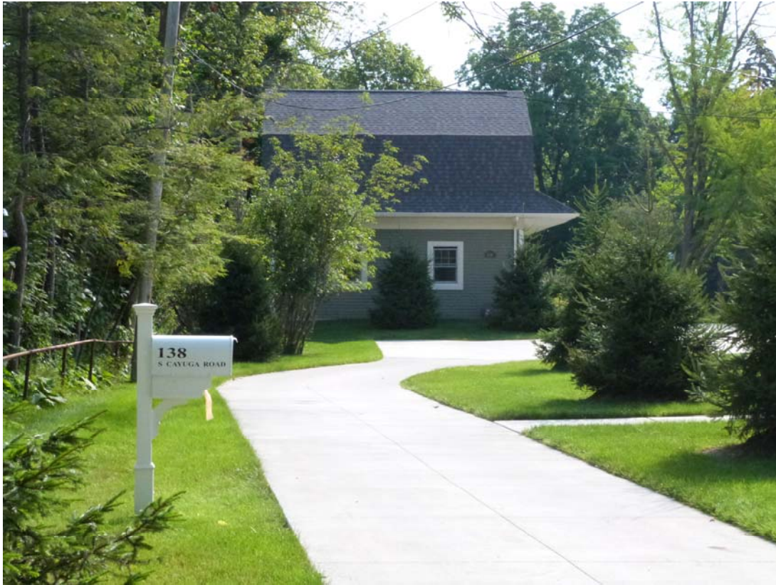
Photo #1: Overview looking east
