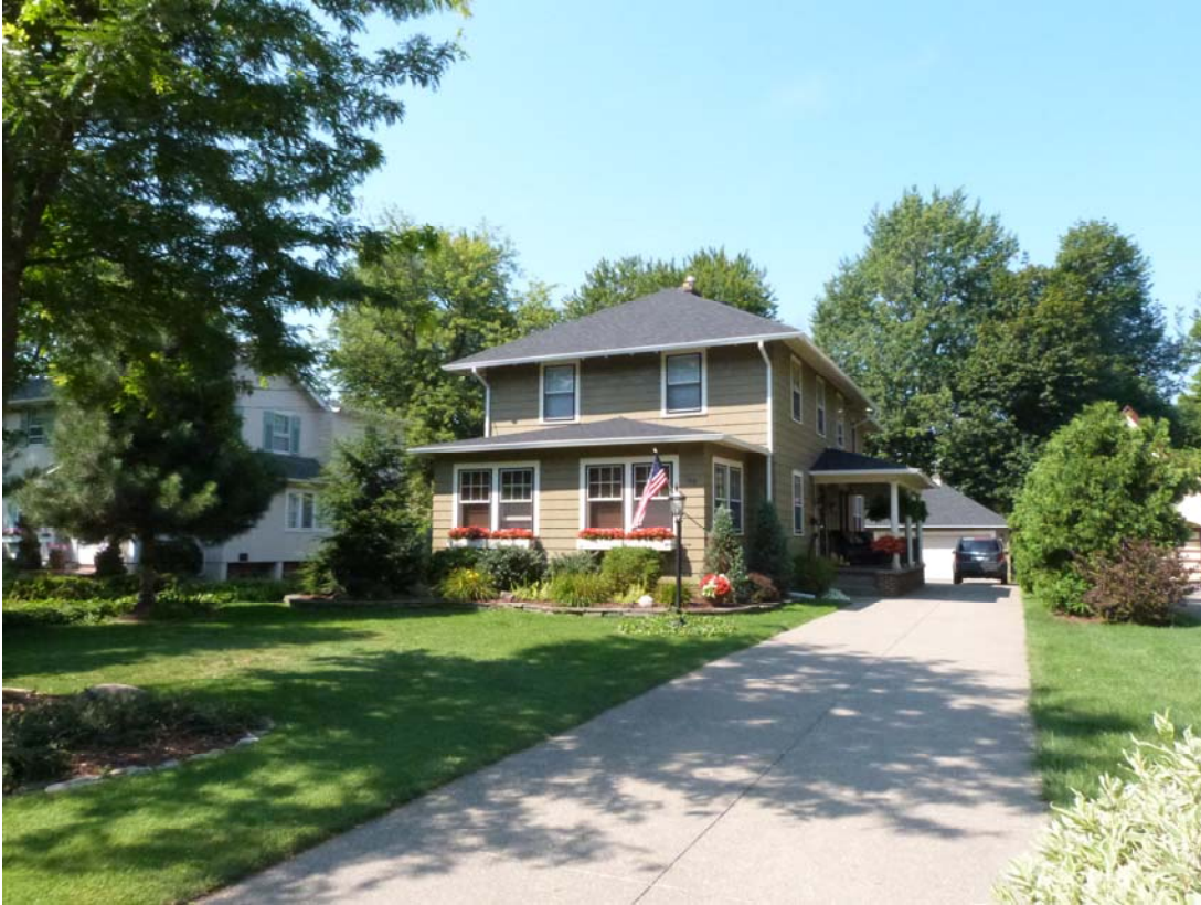
Photo #1: Overview looking southwest
