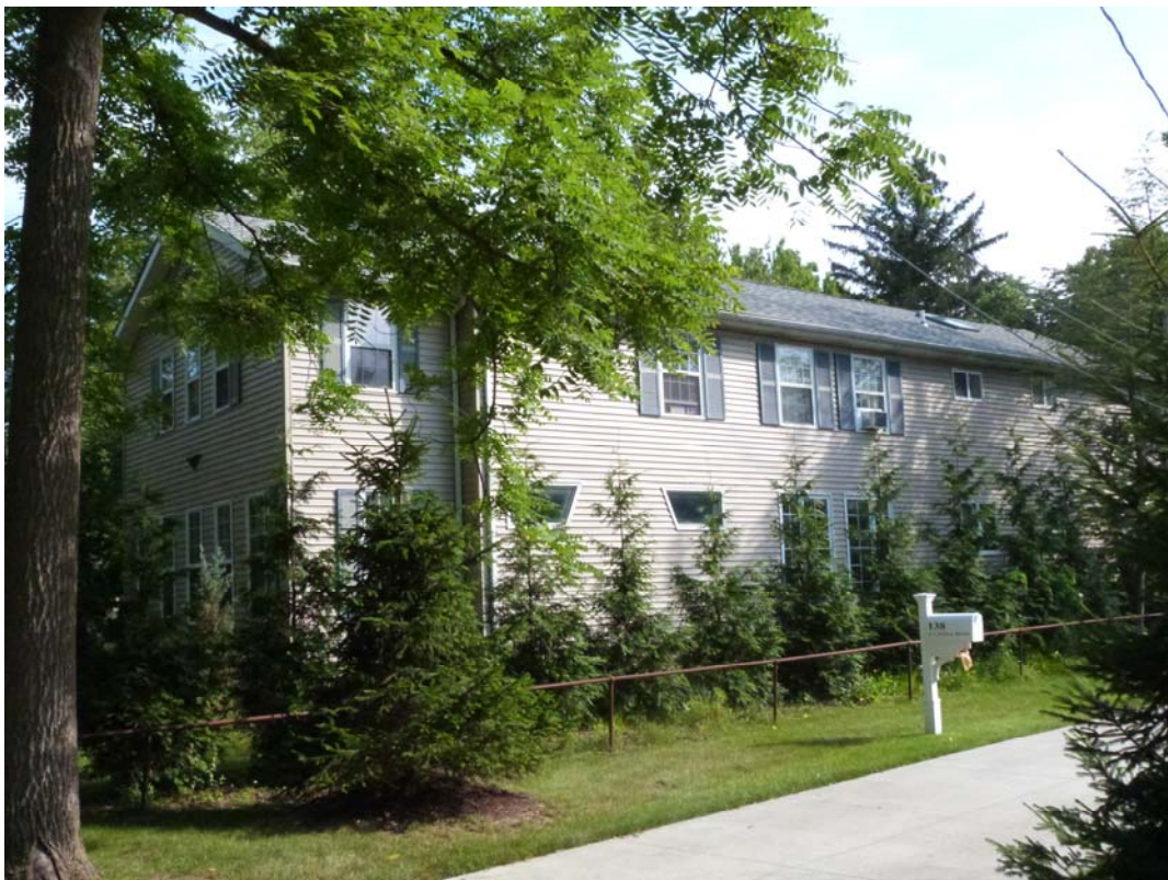
Photo #2: Looking northeast
