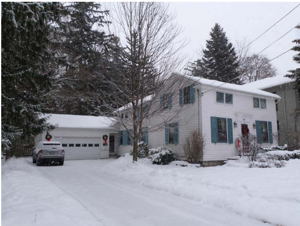
Photo #1: Overview looking southeast
