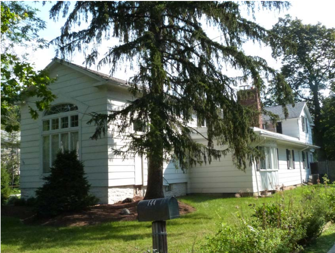
Photo #2: Closer view, looking northeast
