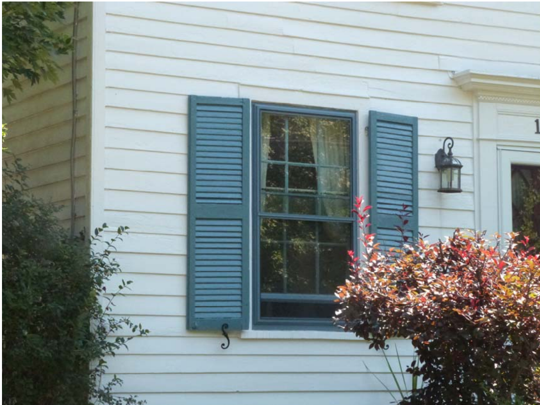
Photo #3: Detail view of wood window and shutters
