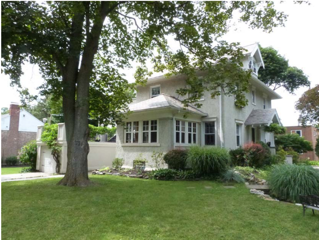
Photo #2: Looking northwest toward house
