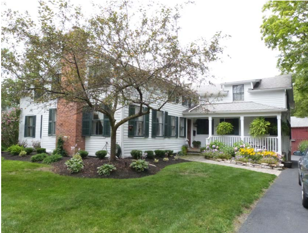
Photo #1: Overview looking west
