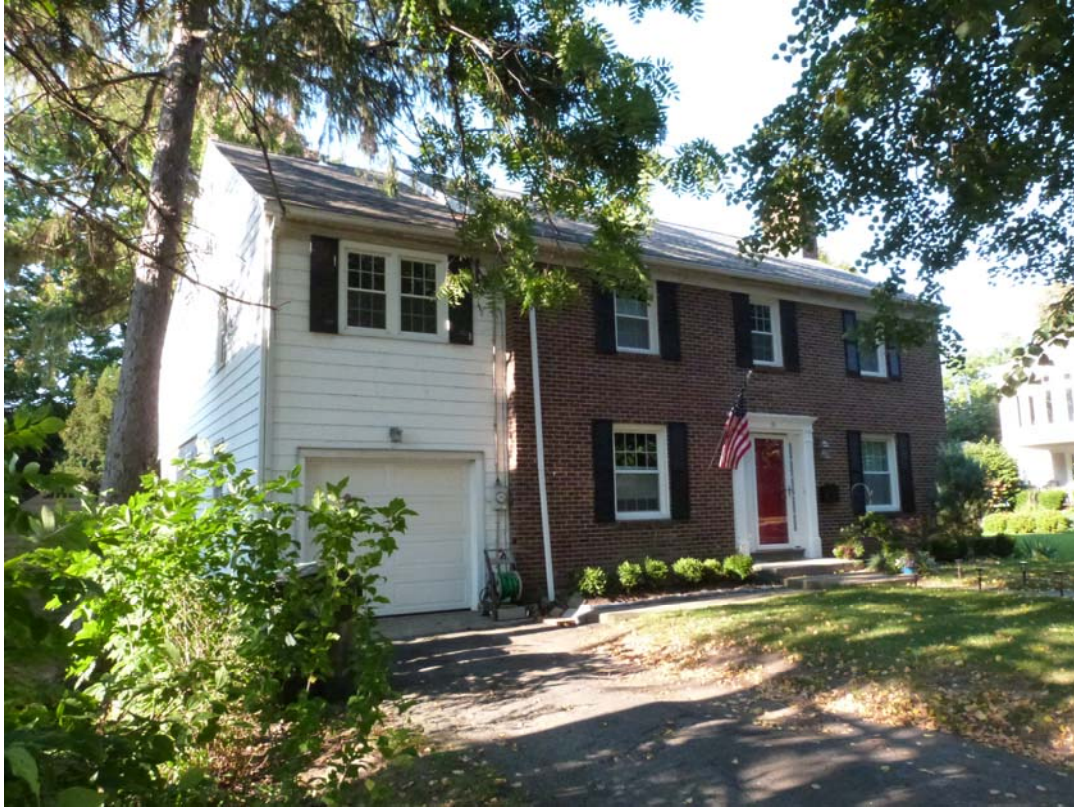
Photo #7: Looking northeast toward rectory.
