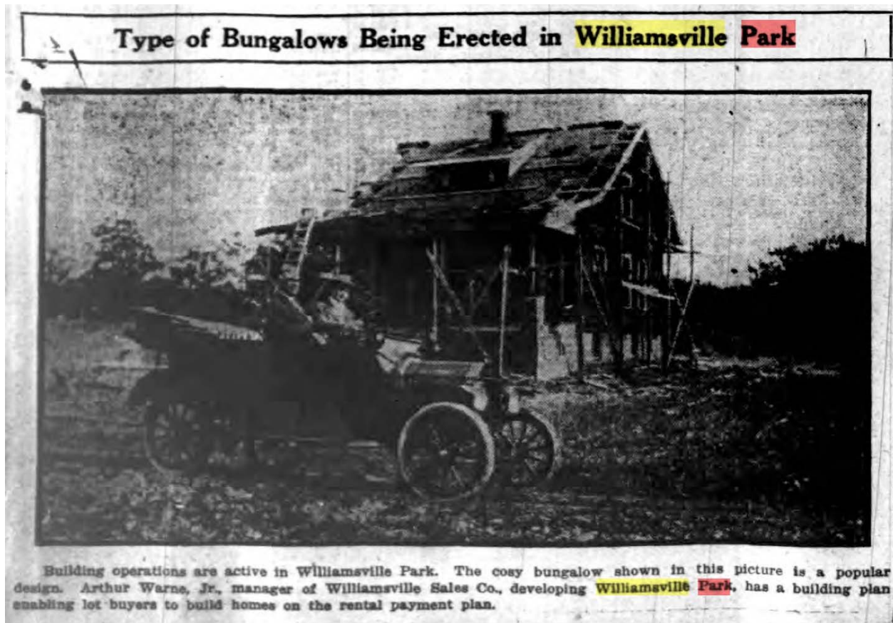
Figure 3-6. A bungalow under construction in Williamsville Park, 1915.
