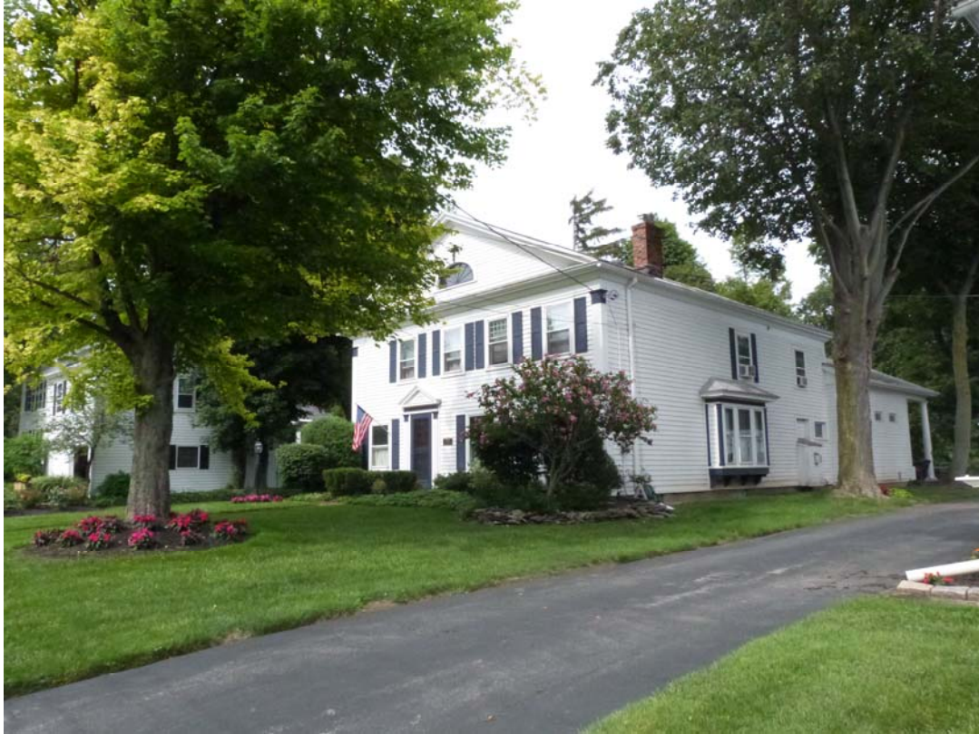
Photo #1: Overview looking northeast
