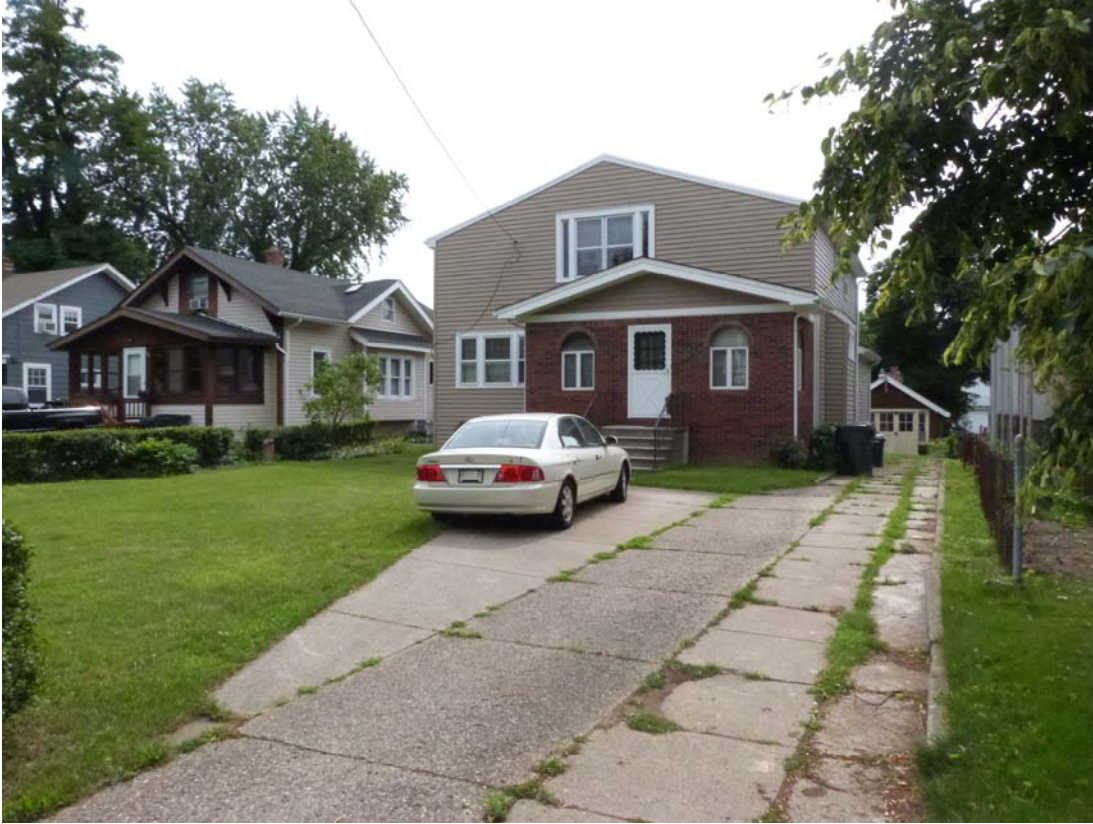
Photo #1: Overview looking southwest
