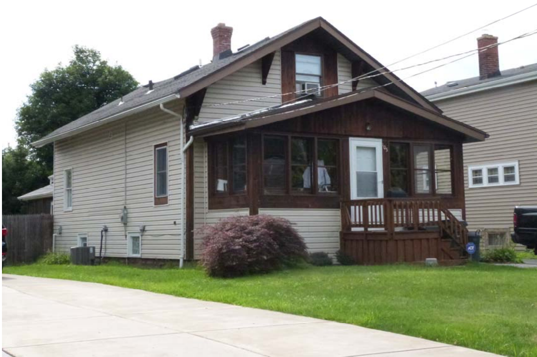
Photo #1: Overview looking northwest
