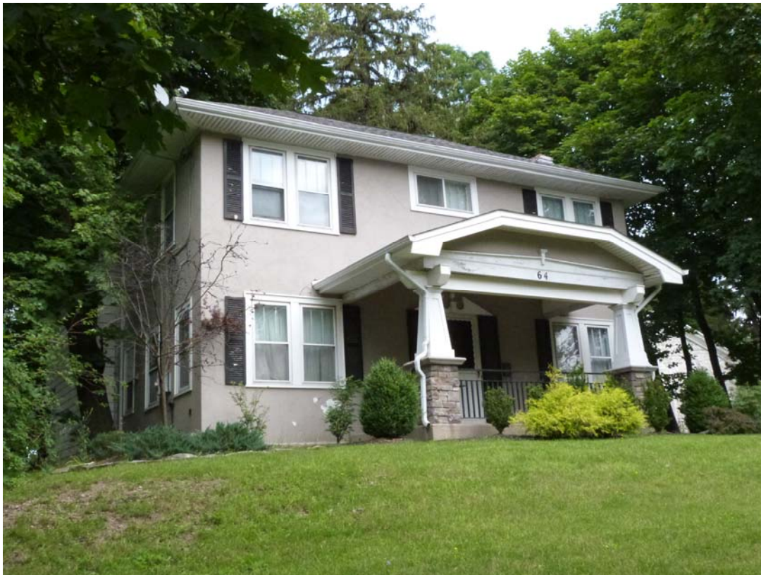
Photo #2: View looking southeast
