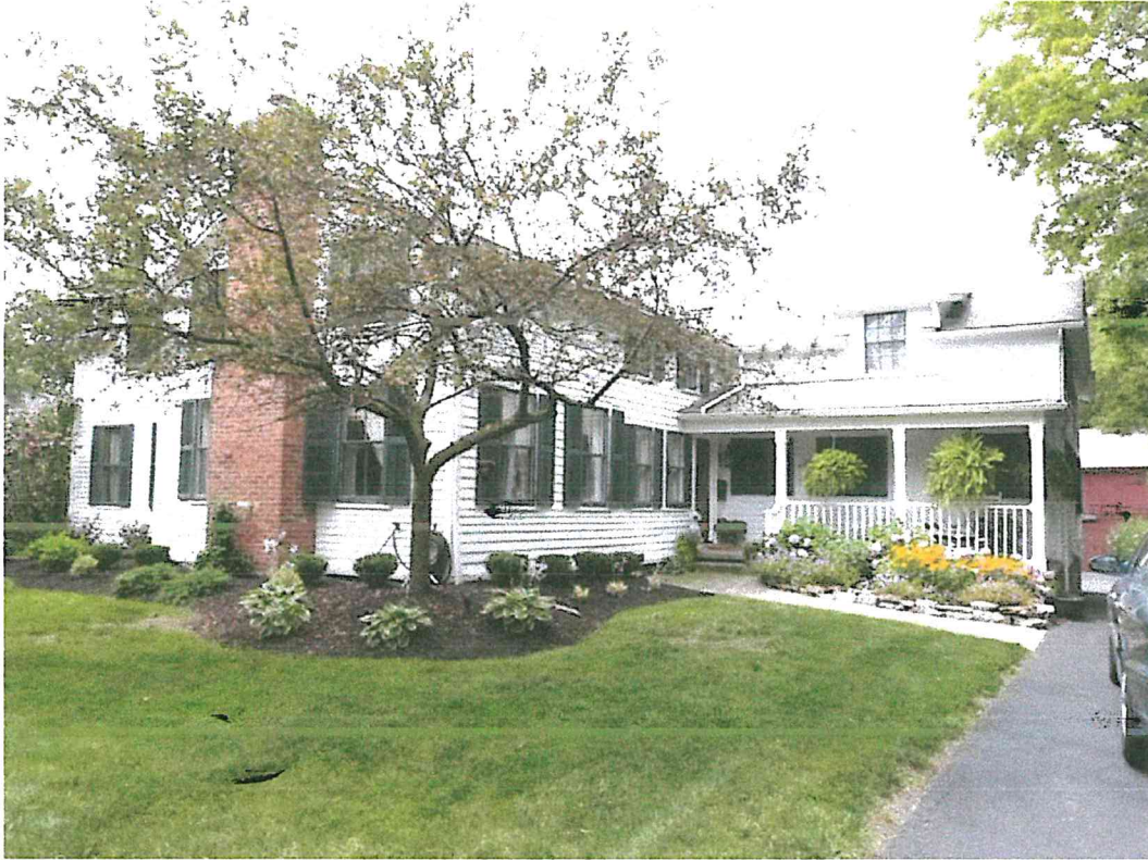
Photo #1: Overview looking west
