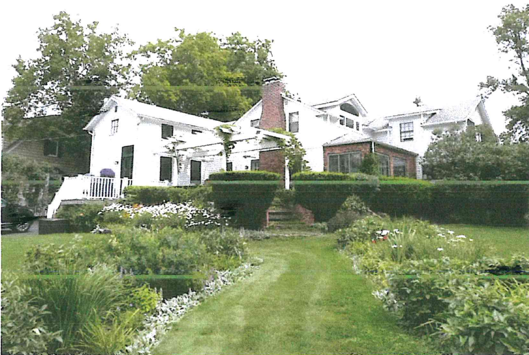
Photo #2: Rear side of house, looking northeast
