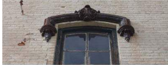
Projecting hood above a window intended to help shed water.
