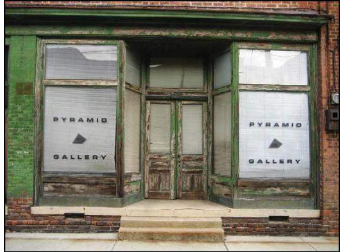
A largely unaltered 19th century storefront including all the elements typical of that era: Display windows, recessed entry, transoms, bulkheads, and signboard above.
