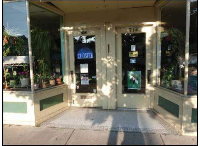
This storefront entry area retains its original wood doors and hardware and display windows over wood bulkheads. Multiple storefronts often share an inset entry.
