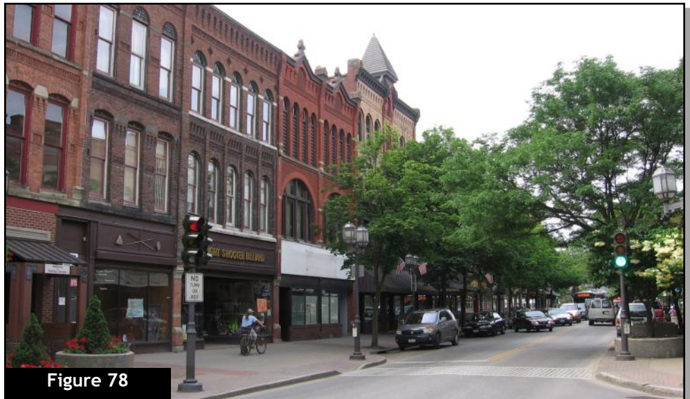
Figure 78 These structures have continuous cornice and trim lines, and provide a high quality rhythm to the streetscape [§ 112-16G(4)(h)].
