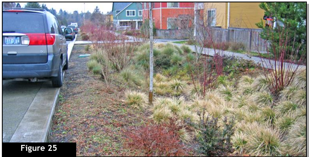
Where appropriate, bioretention areas and bioswales similar to the above may be used to promote the infiltration of storm water. These installations would be appropriate in parking lot medians or in linear strips along drive aisles or behind parking lots in lieu of large, unsightly retention facilities.
