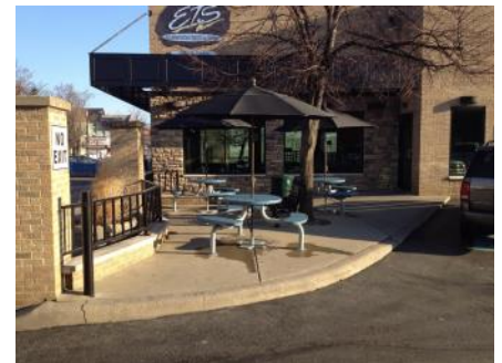
The above represents seating that is removed from the parking facility by a minimum 6" elevation, but lacks the necessary railing.
