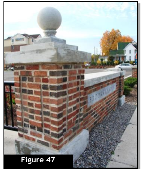
Figure 47 The above structural screen utilizes masonry columns and fencing to provide a visual and physical buffer between a sidewalk and parking area.
